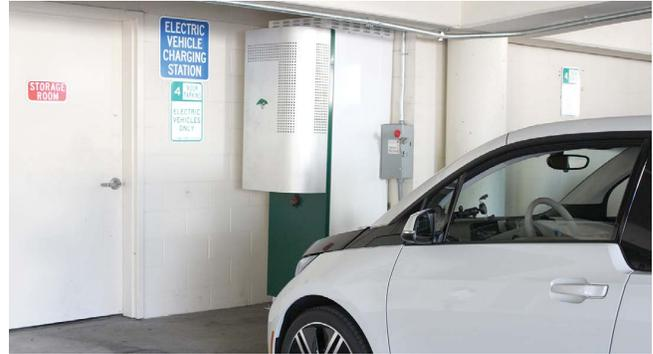
Image depicts Green Charge energy storage system located at the Marshall Street parking garage in downtown Redwood City. The storage system mitigates spikes in power demand due to heavy use of EV chargers and other electrical equipment.
