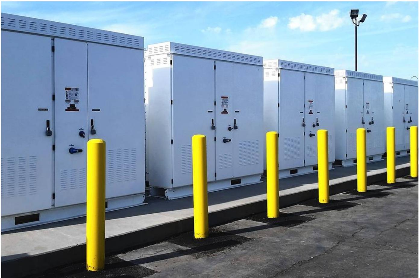
Cargill installed two megawatt-hours of Tesla Motors batteries at its Fresno beef-processing plant to help it save about \$100,000 a year on energy. *Photo: Cargill*
