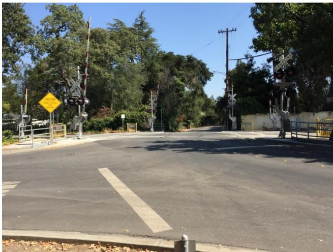
The 4-quadrant gate system provides a higher level of safety since gates are installed across all roadway lanes which prevents aggressive drivers from entering the rail corridor. Since the 4-quadrant gate system does not allow cars to physically enter the rail corridor, it is an approved FRA Supplemental Safety Measure which qualified the Fair Oaks Lane crossing for a Quiet Zone.
