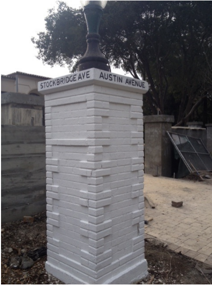
Street pillar refurbished
